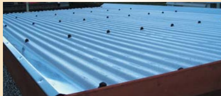
One piece front-to-rear steel roof sheets No joint to leak Anti-condensation coating
