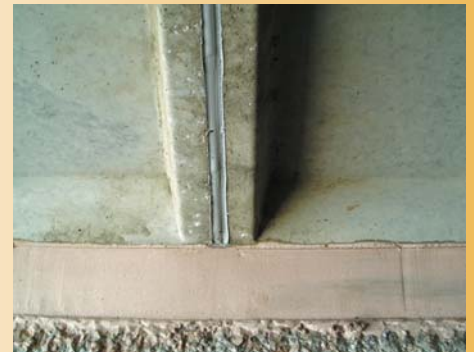
Sand and cement fillet between base and walls, plus mastic sealed panels Prevent water getting beneath or between panels
